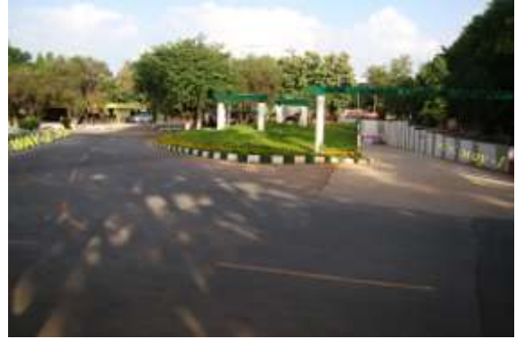
Newly constructed underpass
