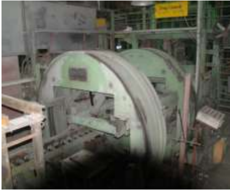
Newly replaced Drag Conveyor
